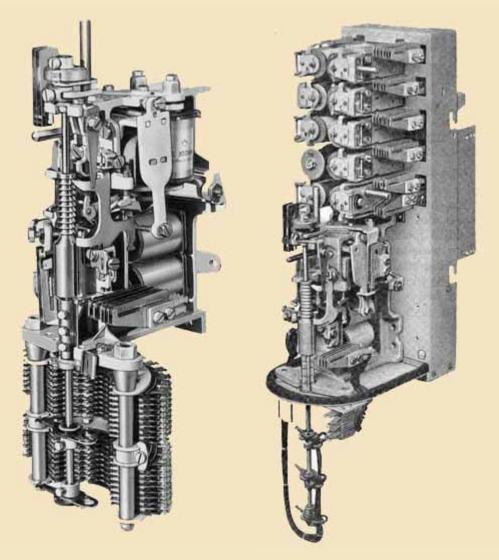
Left: Automatic Electric Belgium step switch, late 1940s. Note the magnets have been moved to
